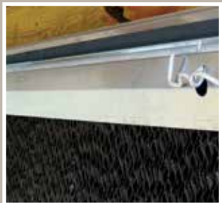
The spray bar bracket and water deflector insure pads are uniformly wet.
