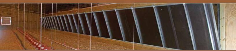
Tunnel inlets help to eliminate dead zone areas created by curtain sidewalls and curtain pockets. The tunnel inlet door comes fully assembled and an ultra lightweight, rigid laminate foam panel construction makes for easy installation. All brackets are galvanized for durability and long life.
