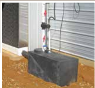
A roto-molded holding tank offers increased water storage capacity.
