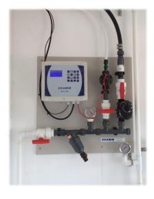
Pre-fabricated manifold panels are available and incorporate a filter and zone solenoids tailored to your site for precise control.
