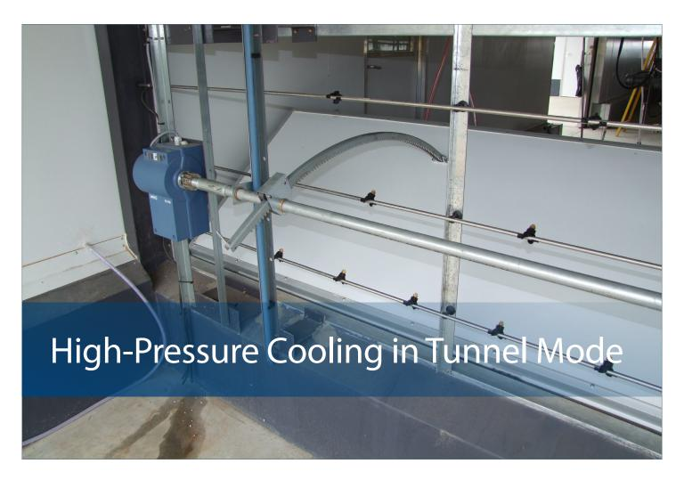
n areas with very high temperatures and low relative humidity it can be an advantage to use high-pressure cooling in tunnel mode.
