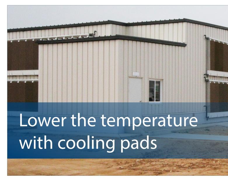
ooling pads can be used for the SKOV Tunnel and Combi-Tunnel systems. The cooling takes place when fresh air is led through cooling pads that are kept damp by sprinkling water. The fresh air is cooled when it absorbs water vapour from the cooling pads.
